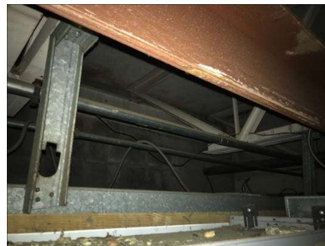
Overhang Air Sealing – there is no barrier separating the exterior overhang (area beyond metal framing) from the conditioned interior space
