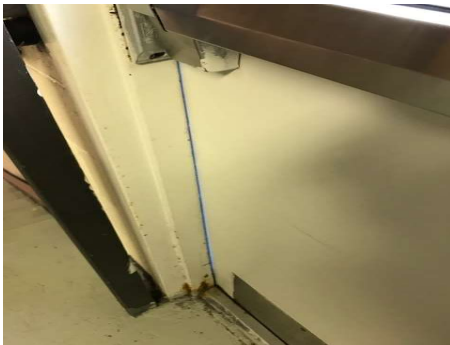
Door Weather Stripping – daylight showing through the sides of the door is a clear indicator that there is not a tight weather stripping seal
