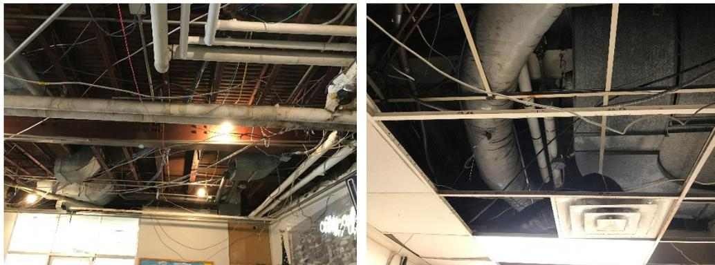
Damaged pipe and valve insulation at the Municipal Building
