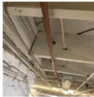
Uninsulated hot water pipe
