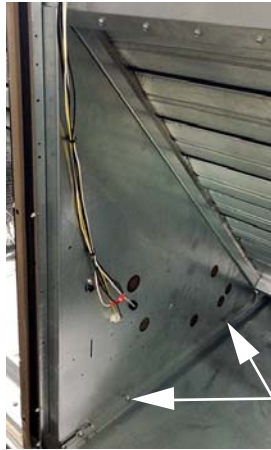
Figure 13 - Attaching the divider to the base
